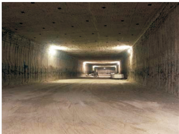
Fig. 1. View of an excavated disposal room in the WIPP underground. These are approximately 4 m high, 10 m wide and 100 m long.
